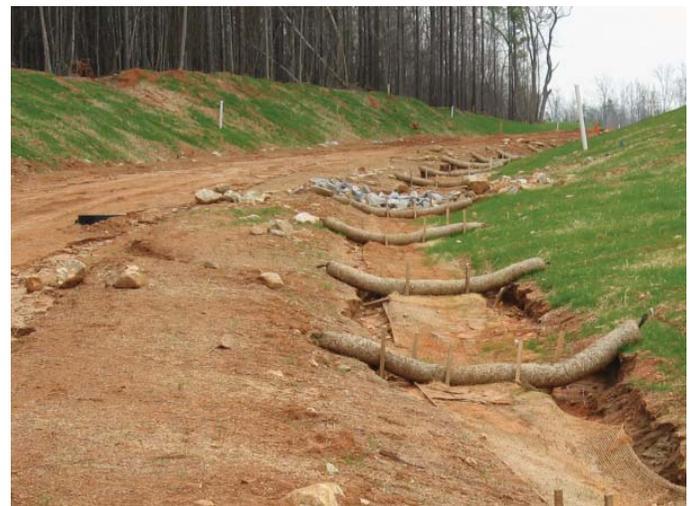
**Figure 6.** An example of improperly installed FCDs and ditch liner. The liner was not extended up the sides of the ditch, and the FCDs were not stapled into the ground. As a result, erosion occurred under the FCDs on the edges of the liner.
