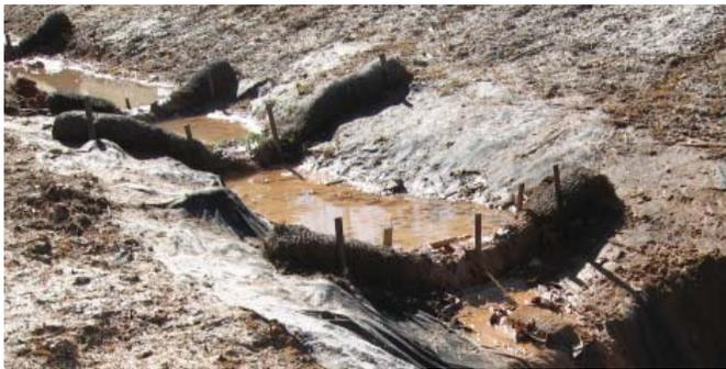
Figure 2. An example of an installed FCD system pooling water in a ditch line.
