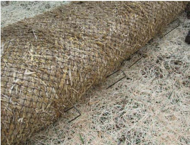
**Figure 4.** Example of how to install FCDs by stapling them to the ground through the netting on both sides. Staples have not been fully inserted into the soil in order to see their placement.
