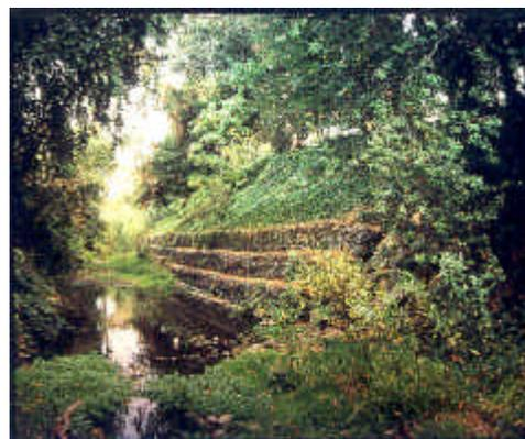
Figure 1. Gabion baskets installed for slope stabilization along a stream
