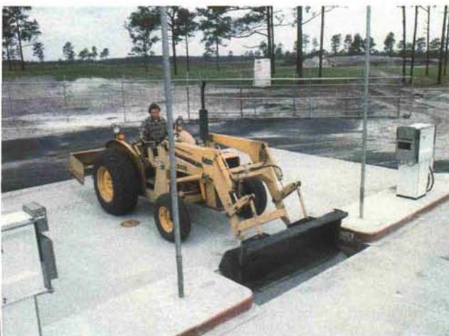
*(Left) Equipment service island — located so that each piece can be serviced and cleaned in the same location. Note the large catch basin for collecting debris from clean-up.*
